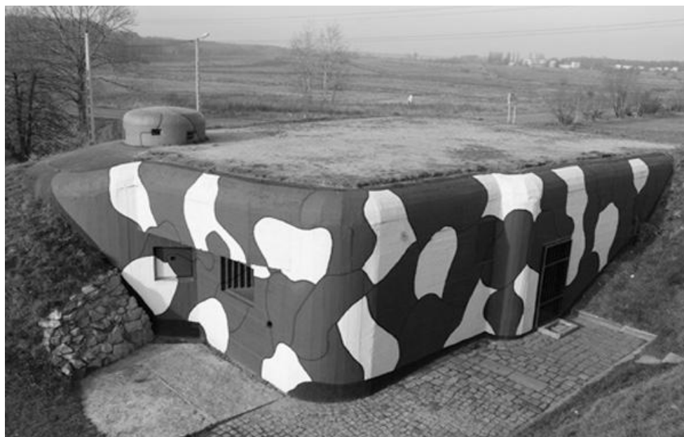
PHOTOGRAPHY 1. First of the renewed bunkers of FA „Śląsk” – Polish battle pillbox no. 52 in Dobieszowice Source: www.profort.org.pl (10.06.2011).
